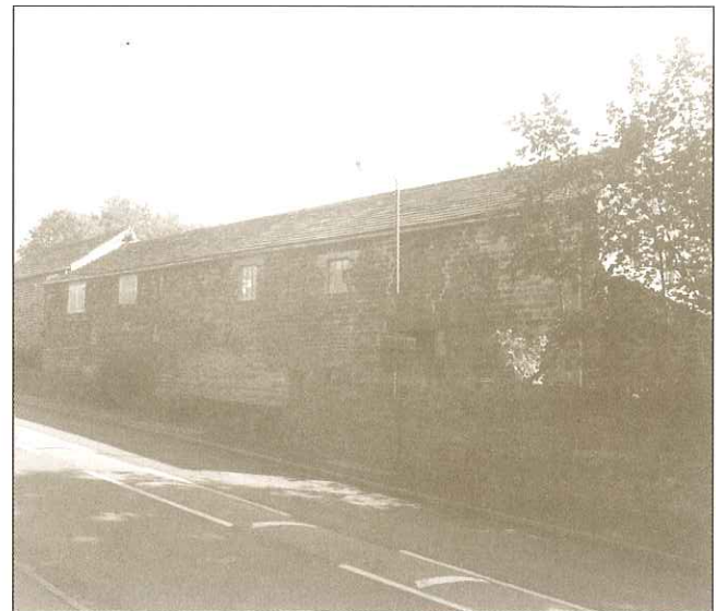
View of Aston End Barns from Green Lane
