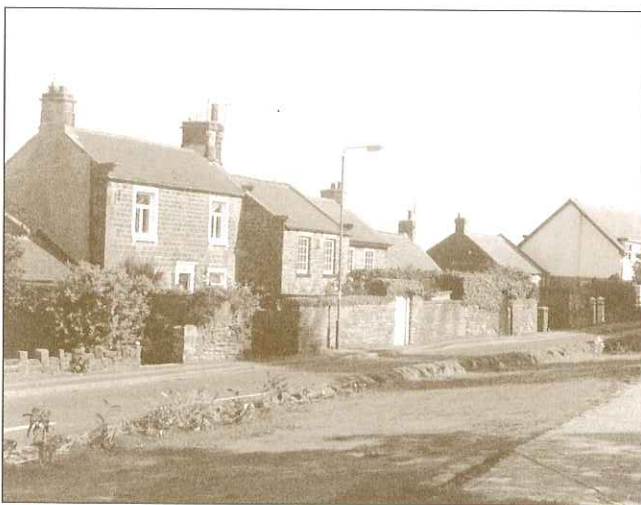
View along Eckington Road
